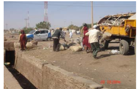
Cleaning drainage canal at Kosti
