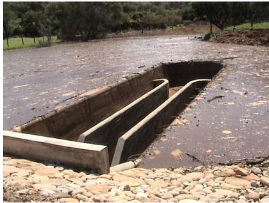
Figure 2. Sedimentation Basin in the Santa Ana River Basin, Calderas, Bolivia
