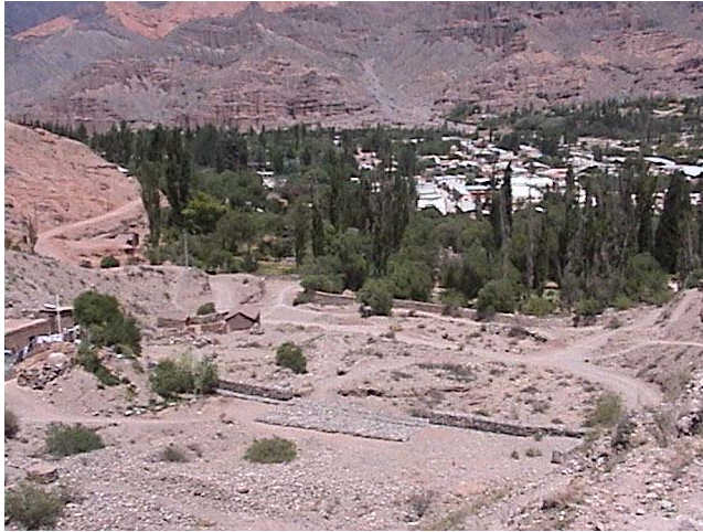
Figure 5. Piedmont erosion control structures in Tilcara, Jujuy.
