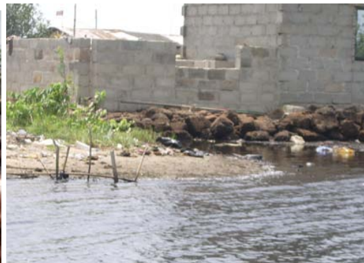
Fig 19- Roots of the Rhizophora used as base to check against tides
