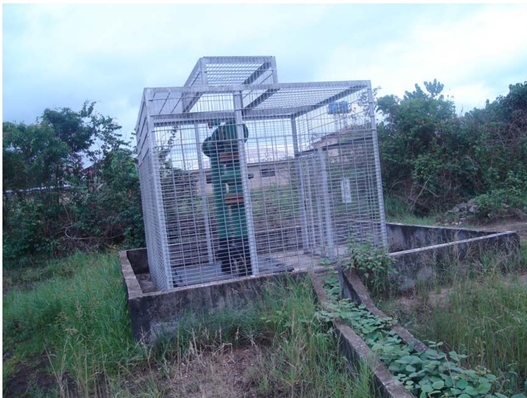
Plate 4: A “Riser” receives and stabilizes pressure of fluids in the oil and gas industry. It brings it down at a point and sends it out at a higher pressure or vice versa as appropriate.
