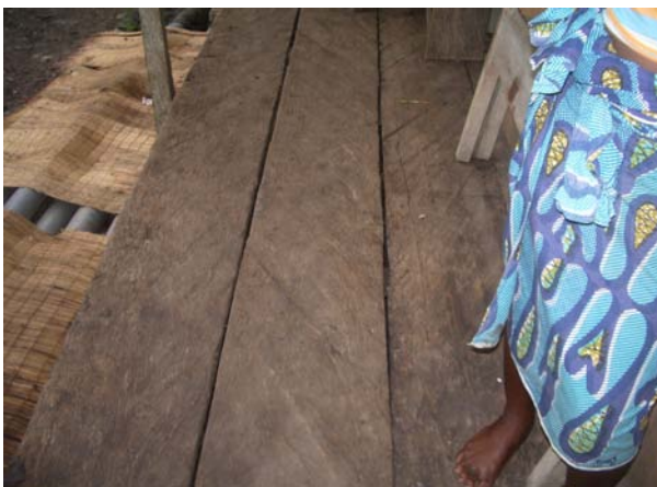
Fig 16-Floor of a house made of sekele
