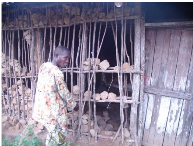
Fig 11 Mangrove Stem used as Skeleton of Houses.
