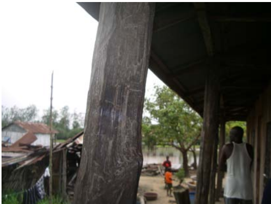
Fig 34(a) & (b)-Red Mangrove used for building support; Being dried for use as pillars
