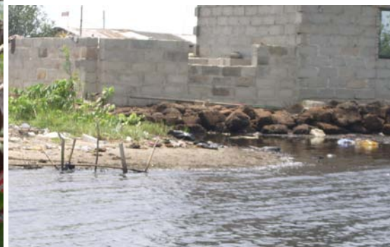
Fig. 13- Roots of the mangrove used as base for their houses
