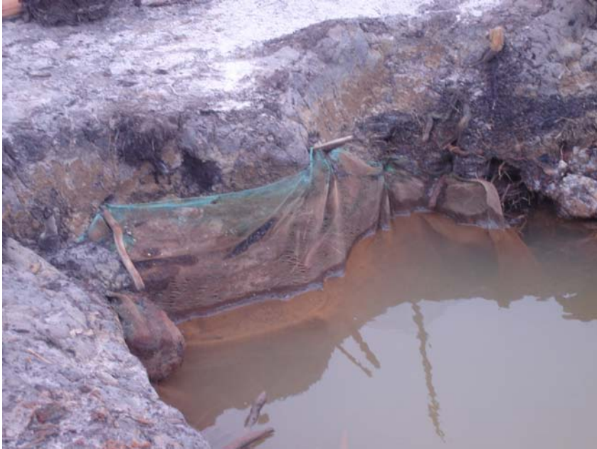
Plate 22: detail of chikoko use in fishpond construction
