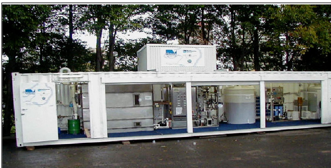
Figure 2.1: Portable WWTW in 12 metre shipping container used for sewer-mining Melbourne, Australia. (Mallia, 2003).
