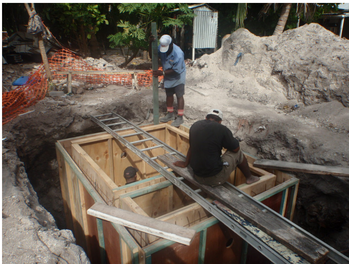
Figure 5 Contractor positioning the conventional Septic Tank mould at the demonstration community in Ewa. 22/02/2011.
