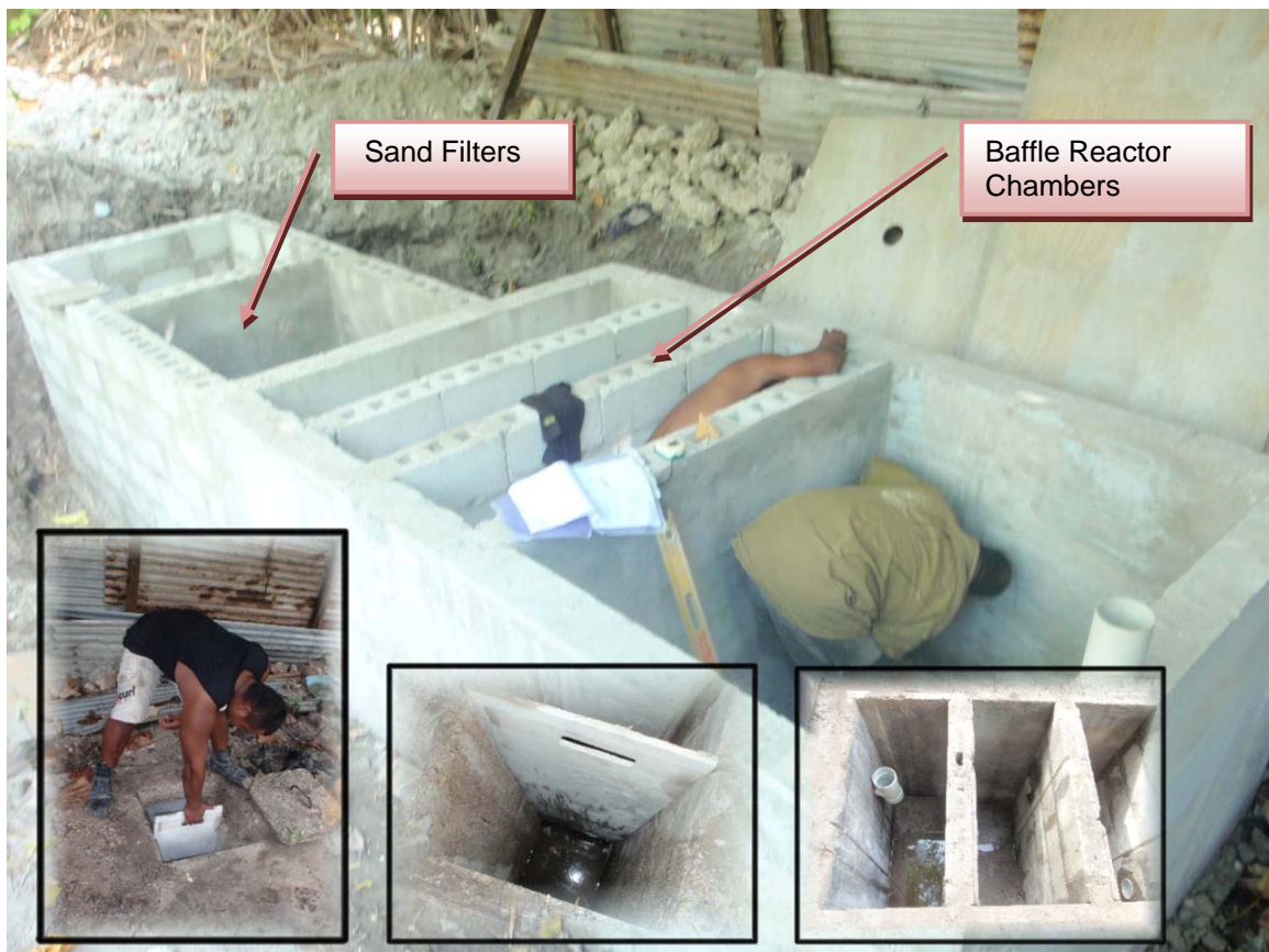
Figure 8 Prototype #2: Improved Septic Tank (Anaerobic Baffled Reactors) with Sand Filter as secondary treatment to improve the wastewater effluent prior Irrigation.
