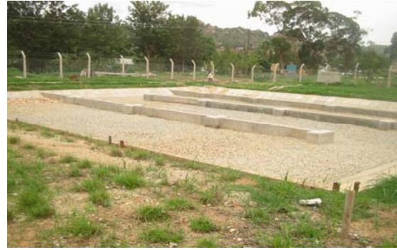
Fig. 3: Constructed wetland replaced the pond
