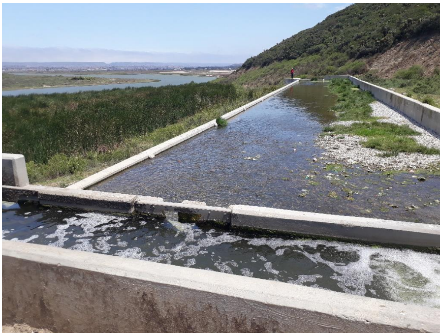
Figure 5. Hard engineering solutions have been established on the Motherwell side of the estuary to control solid waste entering the estuary through the Motherwell canal. Here, wastewater from the canal is directed through a biological filter before entering the river.
