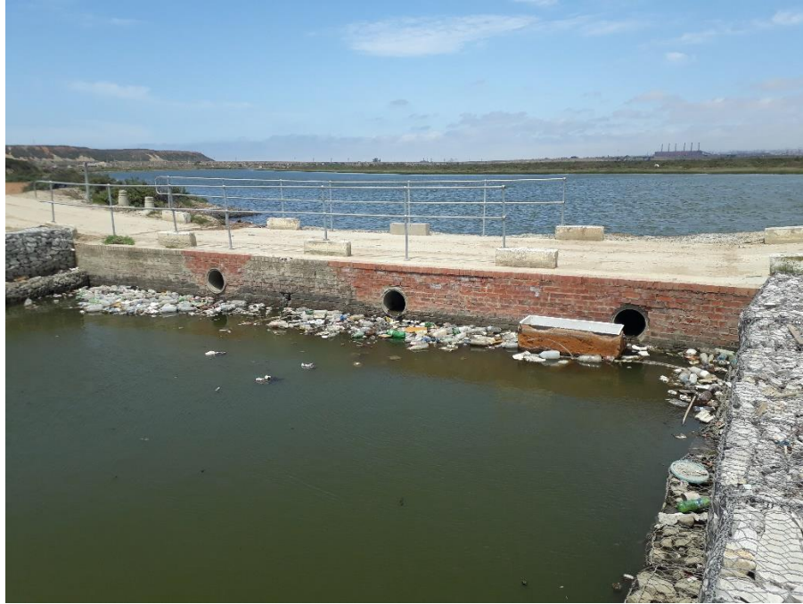
Figure 6. Plastics and other floating waste is collected in a litter trap before water from the Motherwell canal enters the Swartkops estuary.
