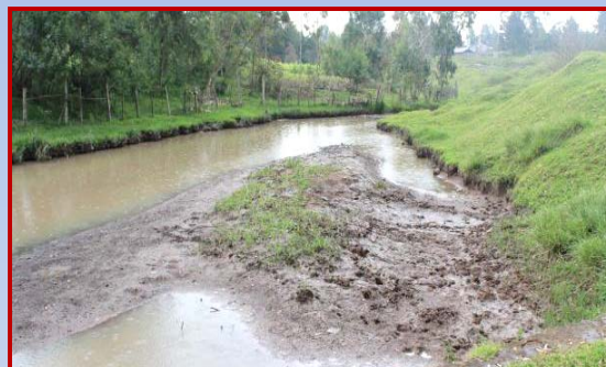
Sediment filled water intake
