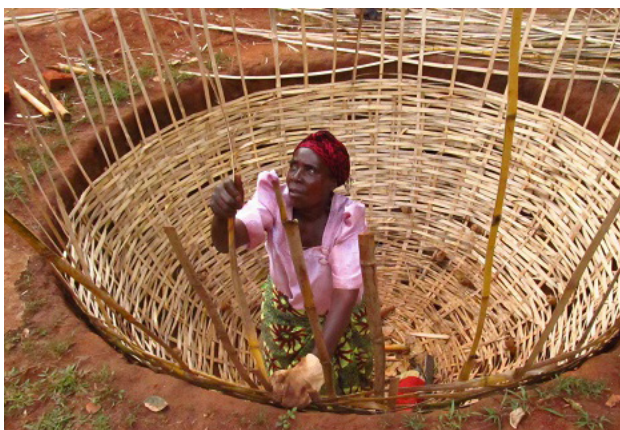
Bamboo-based biogas system are among the most affordable versions in India and Uganda. a) Traditional weaving skills are a basis for bamboo-reinforced biogas domes and can provide additional income for women; b) Clean gas is led into the kitchen to a gas stove for cooking. Photo credit for the left image: © WECF
