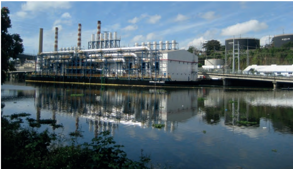
Figure 44: Natural gas fuelled power barge for generation of electricity moored in the city centre of Santa Domingo and supplied by gas from the Andres LNG import terminal and regasification plant
