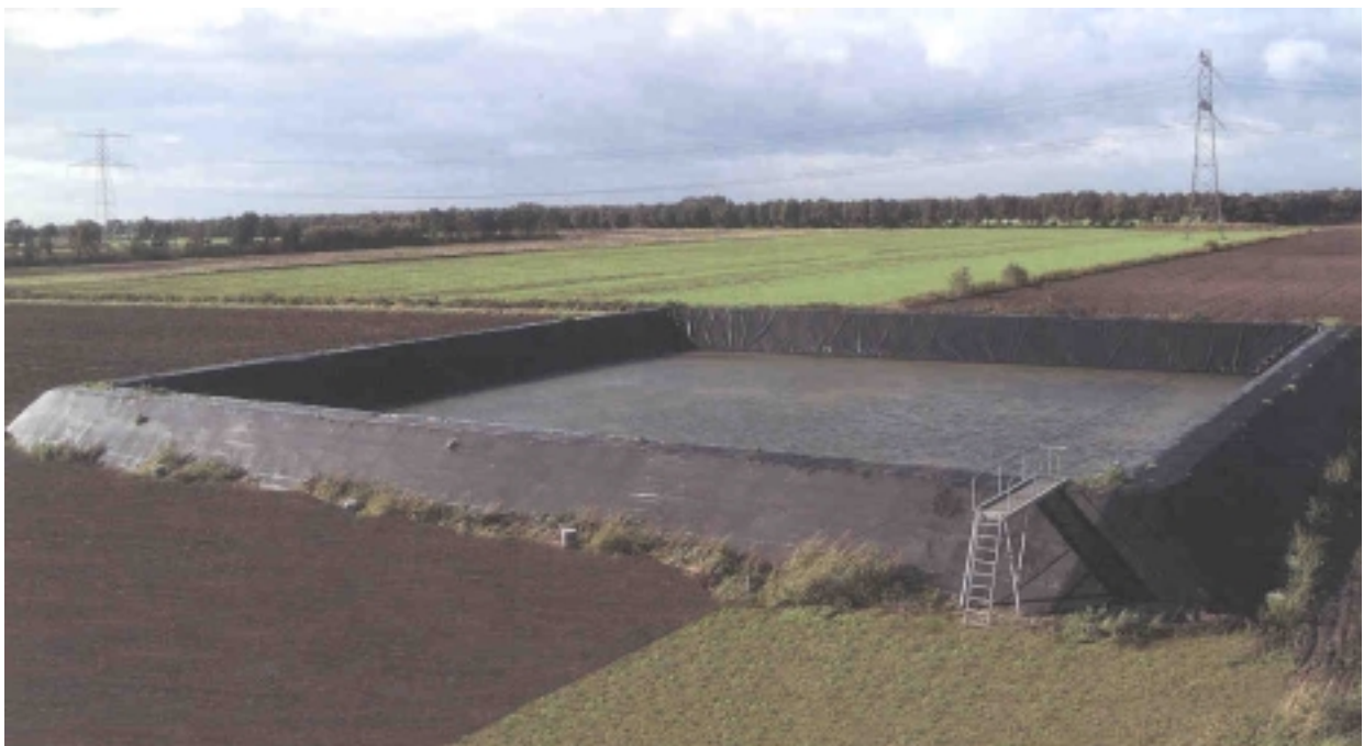
Picture 4 Simple lagoons like this provides a cheap way of storing livestock manure.
