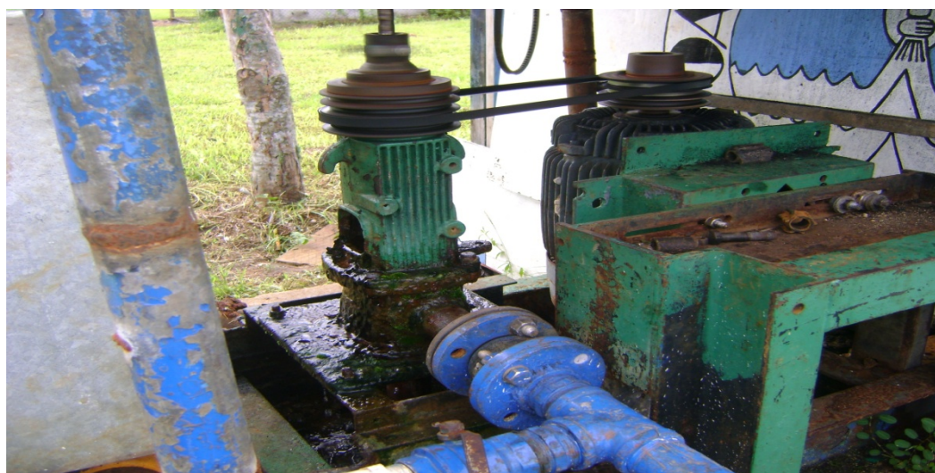
Figure 12 Old infrastructure associated with 70% leakage losses. A key study suggest that old valves may be contributing significantly to losses
