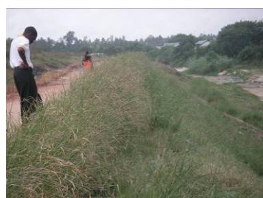
Application of vетiver grass for erosion and leachate control at a landfill site in Dar es Salaam - Tanzania
