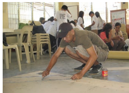
Figure 6. A layer of chipboard is being affixed on the surface of a ½ -inch thick marine plywood.
