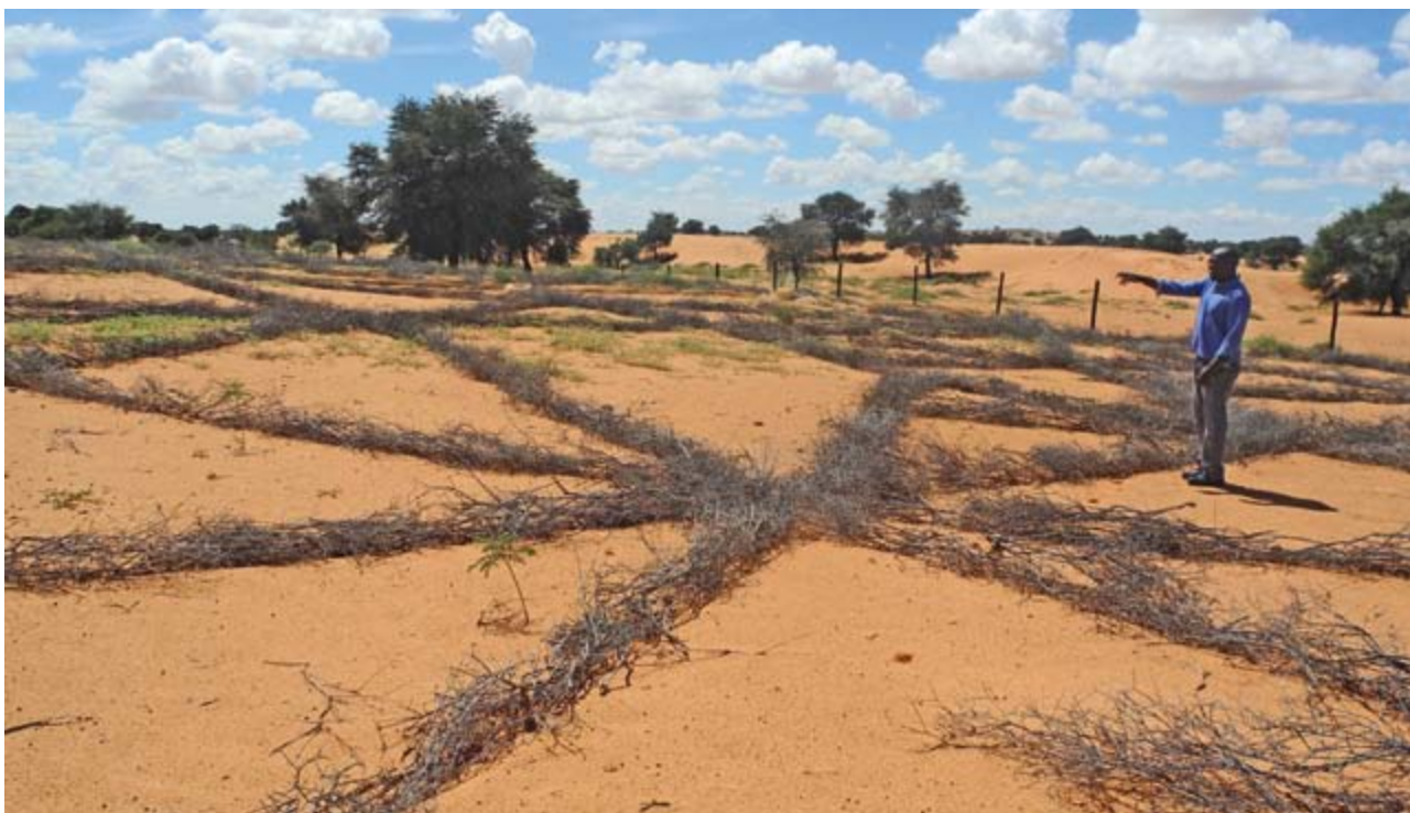
Dune stabilisation demonstration; brush packing with Rhigozum trichotomum branches on the windward flanks of a dune in Khawa, Botswana
