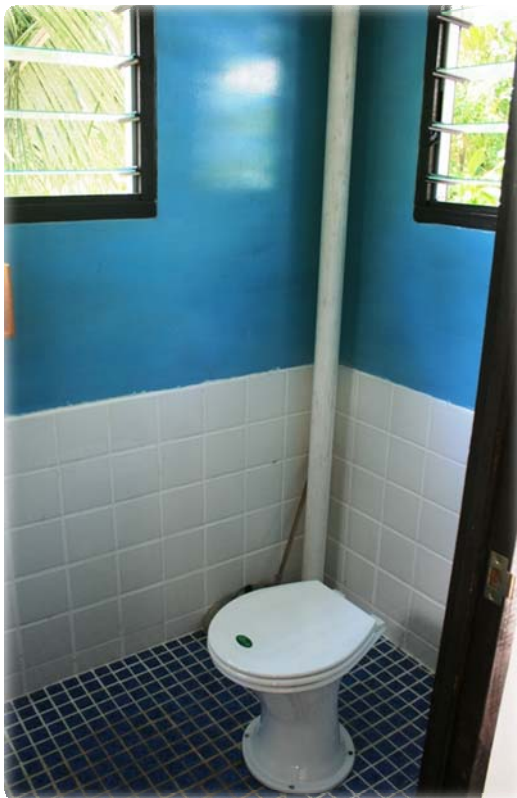
Figure 8 Waterless ecosanitation toilet installed by the project
