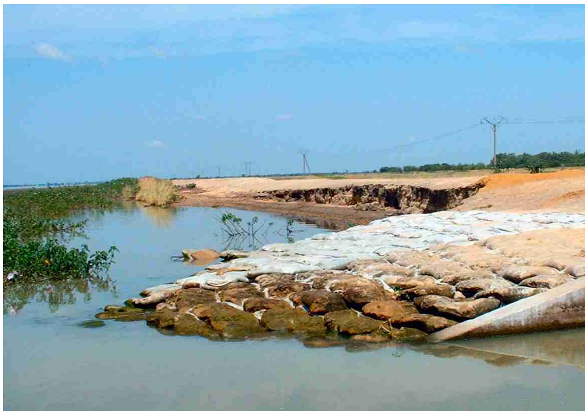
Photo 1 Maga Dam - Erosion and Sand Bag Protection on the Inside Dam Wall
