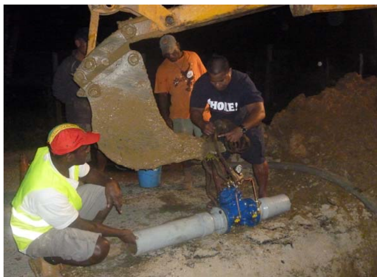
Figure. Leerenson Airen showing the PWD Water Team the installation of PRVs on one of the Luganville System main outlets.
