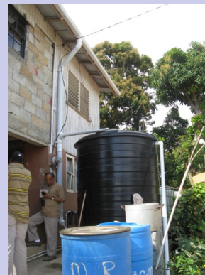
RWH in practice (with old storage tanks alongside), Fond D'or Watershed, St. Lucia
