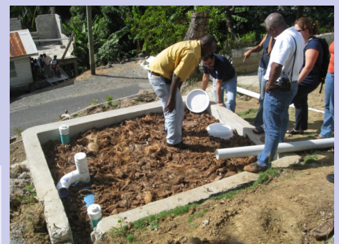
Construction of a wetland wastewater treatment unit
