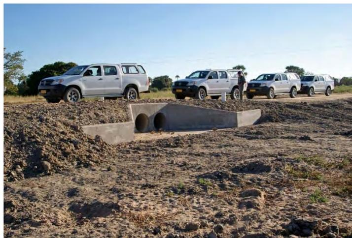
**Figure 3-12 : Culverts constructed in the northern central regions were too small to accommodate flood and storm water**
