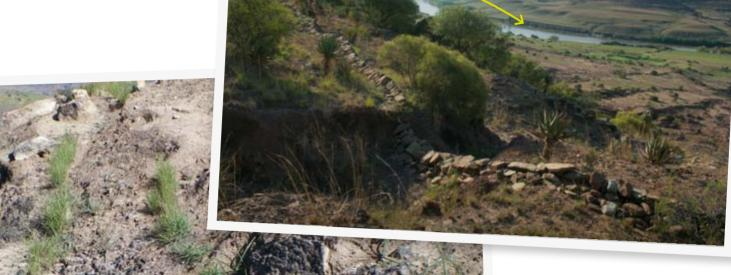
A stone wall that has been built to stop the soil washing away
