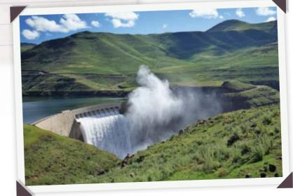
The Katse Dam wall is huge and is made from cement. At the bottom it is more than 60 metres thick. It has to be this thick to hold back the large amount of water behind it.
