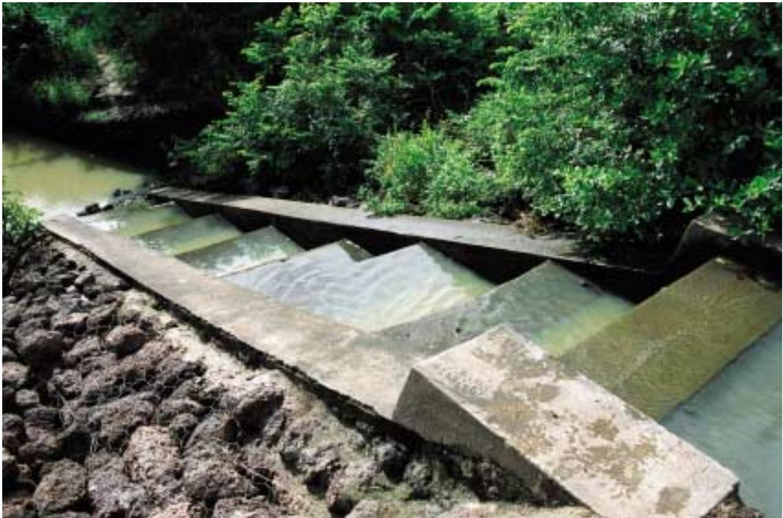
Fish ladder enables fish to migrate beyond irrigation dam (Burkina Faso). Fish ladders are an important infrastructure improvement that can accompany environmental flow releases.
